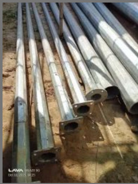
12.5 Meter High Mast Pole
